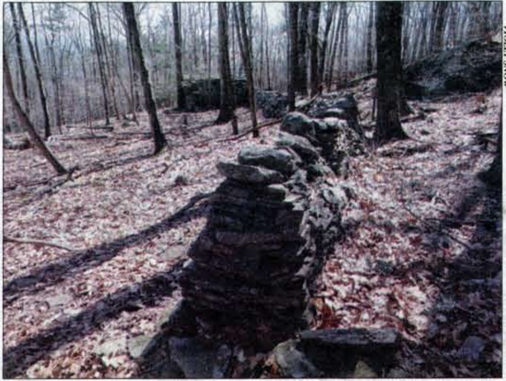
Curving stone wall that ends at the boulder in the background. Note the wall's pyramid shape that adds stability to the structure.
